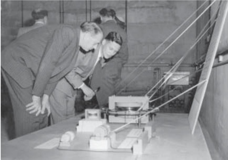
used it to construct and test successfully a model homopolar generator. Mercury, instead of liquid sodium, was used for the contacts.
