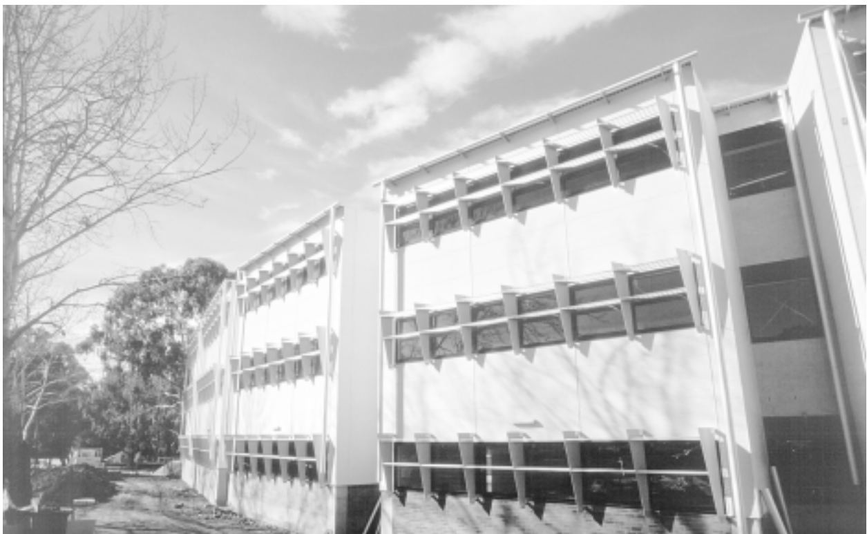
The Innovations Building under construction
